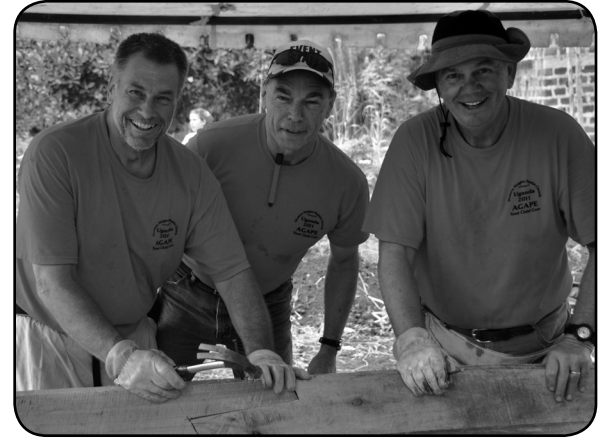
Members of the Western Heights Baptist Church team prepare to roof one of the buildings at Agape Total Childcare Center's new property in Uganda.
