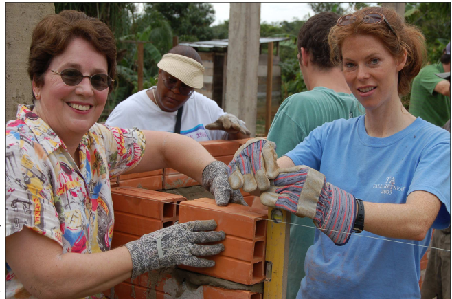
Janet Coppage (left), Phyllis Chappell and Lauren Jones work on building a wall of the new building at the internado.
