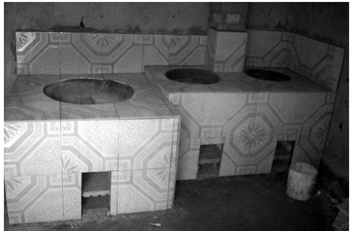
The new kitchen features cookstoves built using the appropriate technology William learned at SIFAT. Community members helped build these stoves and began learning how to make fuel-efficient stoves for their own kitchens.
