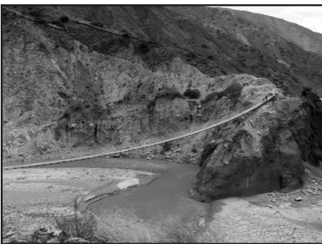
The river is about 100 feet below the bridge. In just a few short weeks, it will fill the valley and make crossing dangerous.
