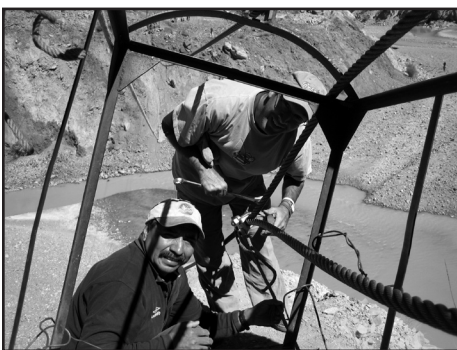
A team member assists Bolivar Sanga, SIFAT's engineer, with attaching the first cable to the gondola to begin stretching it across the river.
