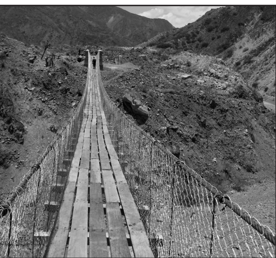
Quesimpuco, Bolivia, SIFAT teams completed a 300-ge to give community members access to the high medical center and boarding home built during ous SIFAT trips. Even during the rainy season, sands now have a safe way to cross the river.
