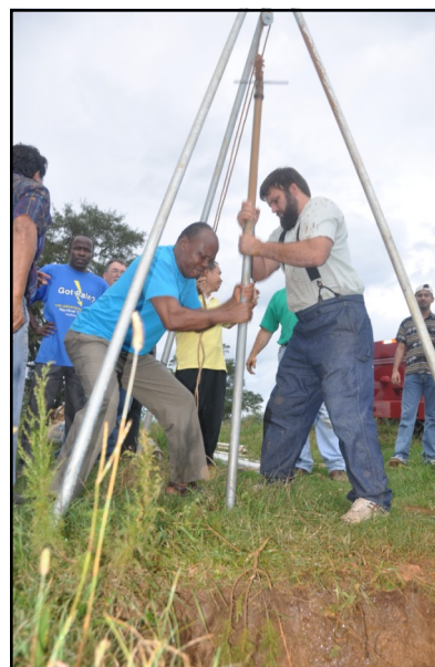
Low tech well drilling
