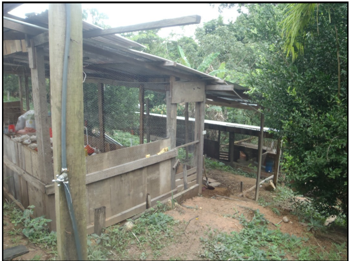
Two chicken houses built on the side of the hill
