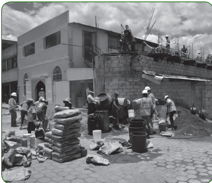
Construction continues in Calderon! In 2016, construction teams will again work with Pastor Raul and Pastora Ruth's church on the addition for classrooms, a kitchen and cafeteria.
