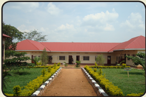
New site in Mukono, 2012
