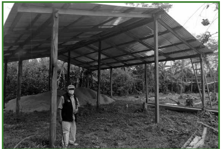
Benjo oversees the building for the chicken farm in Bolivia.
