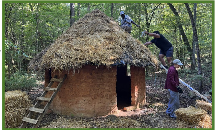
Raphael (on the roof) leads our campus staff in rethatching the roof on one of the Nigeria houses in the Global Village that he led Learn & Serve youth in building on a visit years ago.
