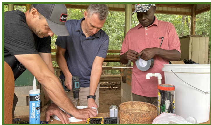
Above: While at SIFAT, Raphael had the opportunity to train friends of SIFAT on biosand water filters, which he learned in SIFAT training and has been using in Nigeria.
